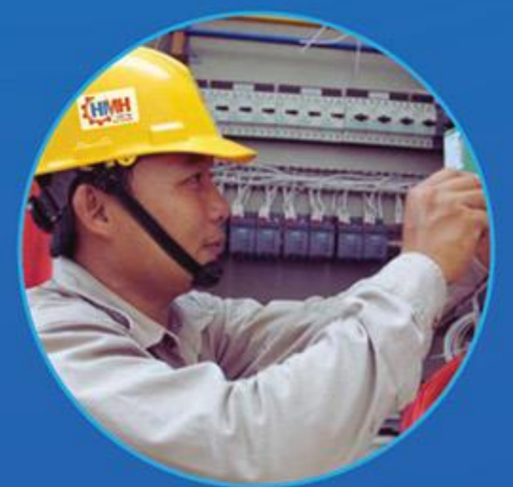
Thi công Construction
