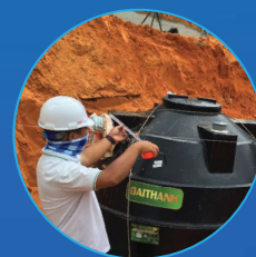
Thi công Construction
